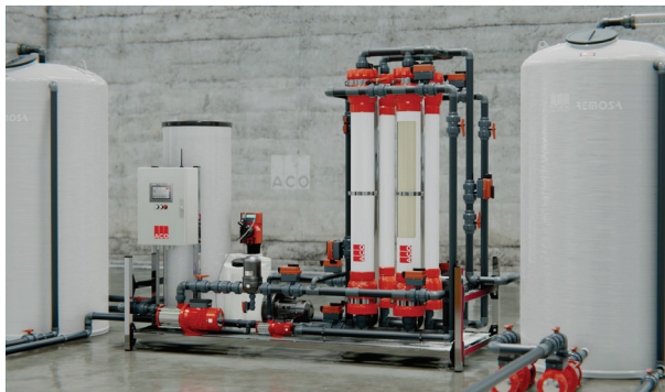
Ultrafiltration (UF) and Reverse Osmosis (RO) systems
