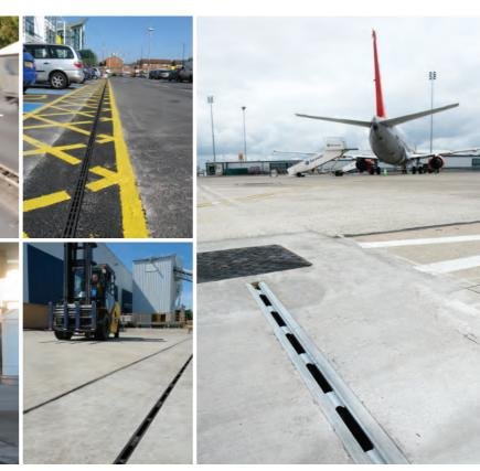
The edge rails are available in three different inlet slot designs: ACO Q-Flow, ACO Q-Guard, and for landscaped areas with block paviours or flags, the ACO Q-Slot galvanised steel edge rail provides a discreet, unobtrusive finish.
