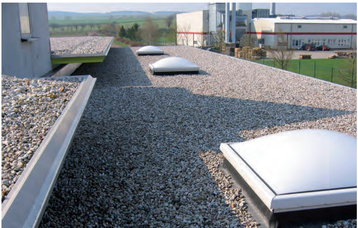
Flat roof with a gravel protection layer
