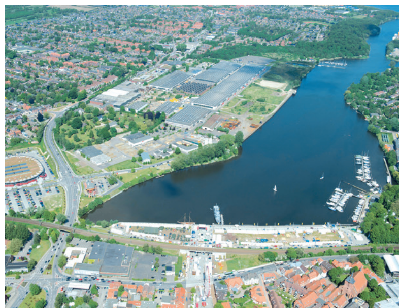
Headquarters of the ACO Group in Rendsburg/Büdelsdorf
